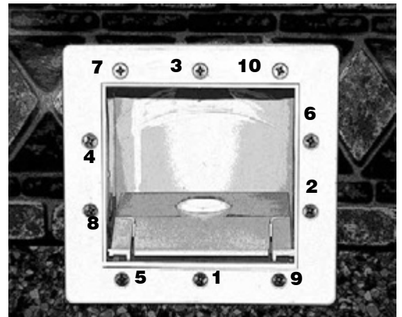
Skimmer faceplate installed w/screw tightening sequence.
